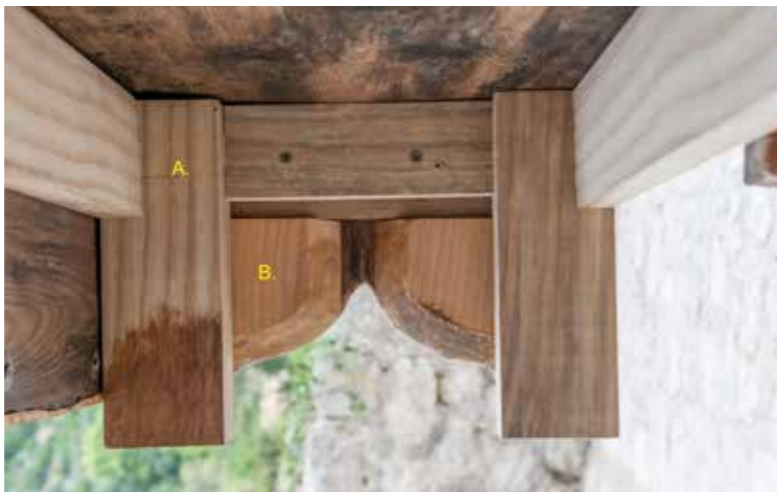
Figure 11 View underneath the bench: A stand made of Accoya wood (A.) now forms the stable base for the bench. The two supporting boards (B.) for the furniture legs can be seen behind the feet of the stand (2016).
