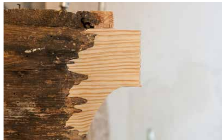
Figure 9 Replacement of missing parts: wooden stick filling with a veneer cover (2014).
