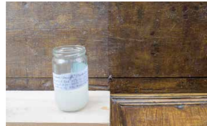
Figure 13 Application of protection varnish: the varnished surface on the right improves the appearance (2018).
